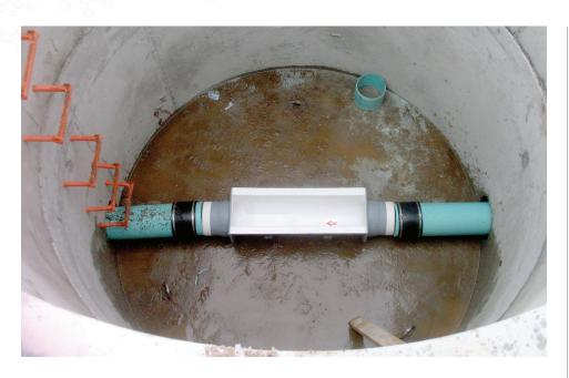
Bulkheads are flat, vertical plates that are chemically bonded (or attached) to the inlet of a HS / H / HL flume approach section or the inlet / outlet of a Palmer-Bowlus flume that provide a surface into which a pipe stub, flange, or caulking collar can be molded to allow the flume to connect to piping.
